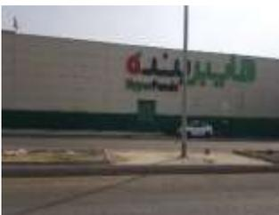
The subject property is a supermarket known as Panda Hypermarket. It is single storey and constructed of reinforced concrete & steel frame structures with painted concrete exterior and interior walls, ceramic tiles flooring and bare ceiling.
