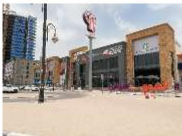
The above property is a single-storey with mezzanine and basement, commercial showroom building constructed mainly of reinforced concrete structure with glass panel, aluminum cladding and brick-stone finish façade; painted concrete exterior wall and glass on aluminum frame main entrance doors.
