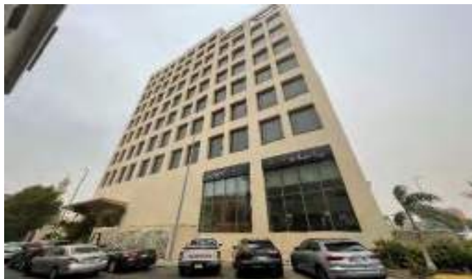
Source: JLL Inspection 2022
