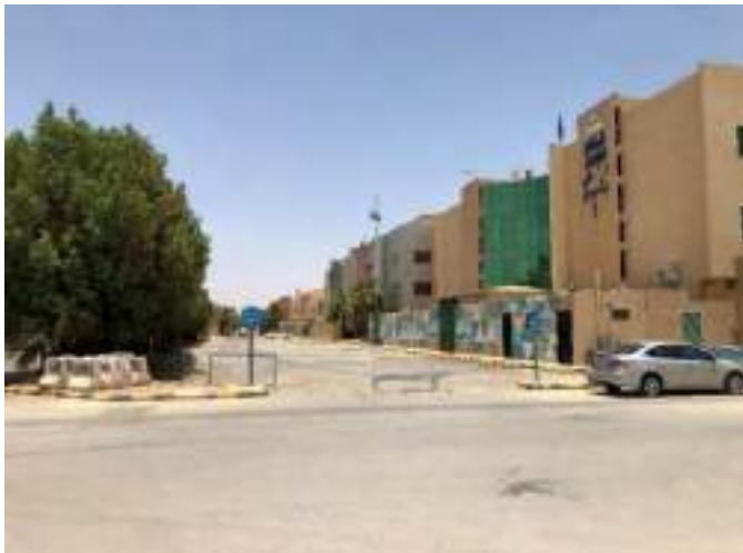
Source: JLL Inspection 2022
