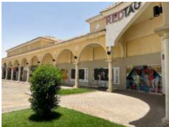
Source: JLL Inspection 2022
