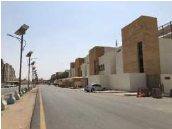
Source: JLL Inspection 2022
