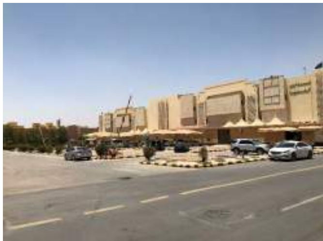
Source: JLL Inspection 2022
