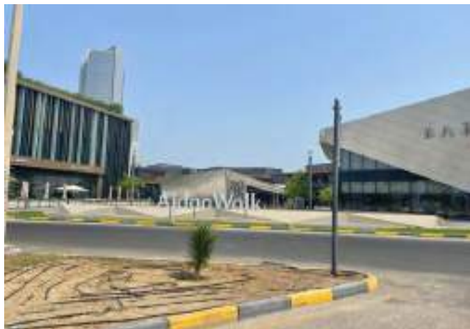
Source: JLL Inspection 2022
