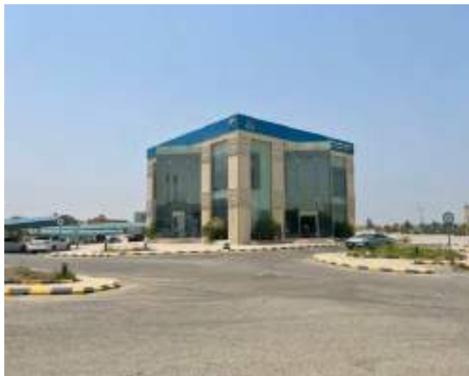
Source: JLL Inspection 2022
