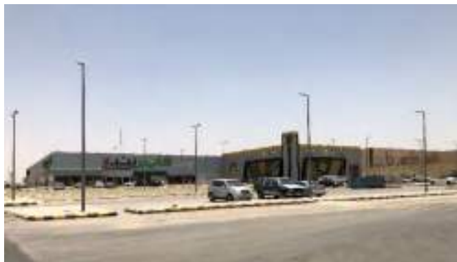
Source: JLL Inspection 2022
