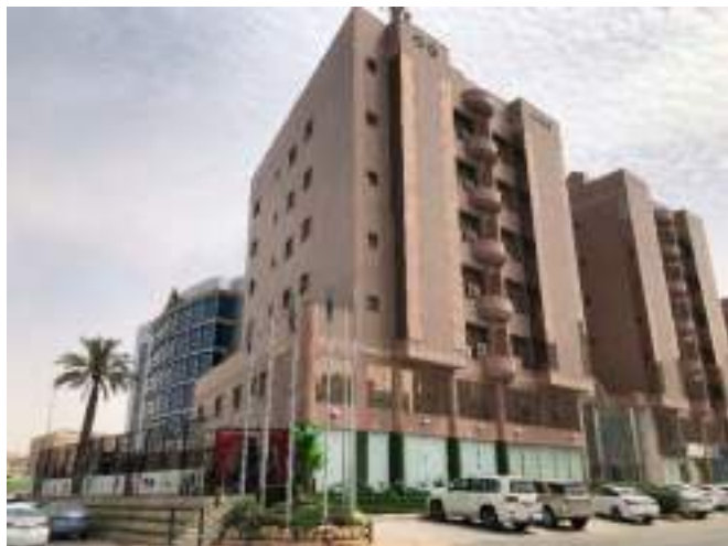
Source: JLL Inspection 2022
