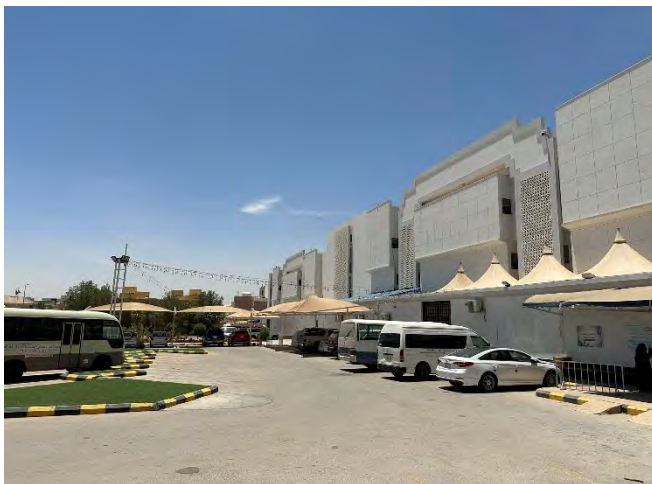
Source: JLL Inspection 2024
