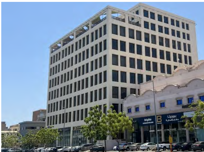
Source: JLL Inspection 2024
