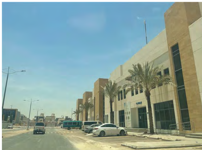
Source: JLL Inspection 2024
