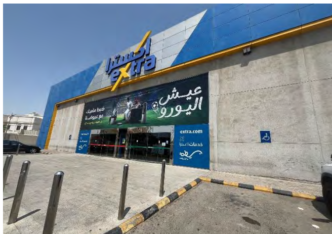
Source: JLL Inspection 2024
