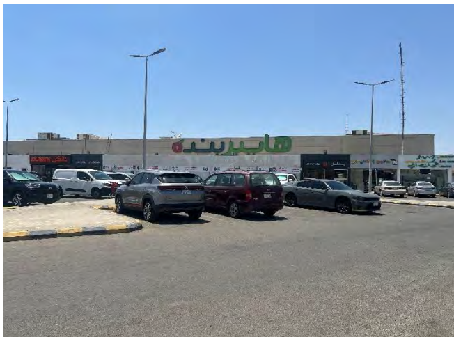
Source: JLL Inspection 2024
