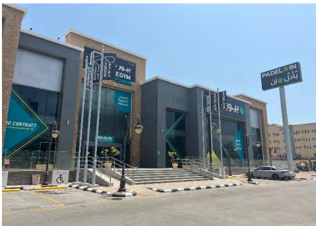
Source: JLL Inspection 2024
