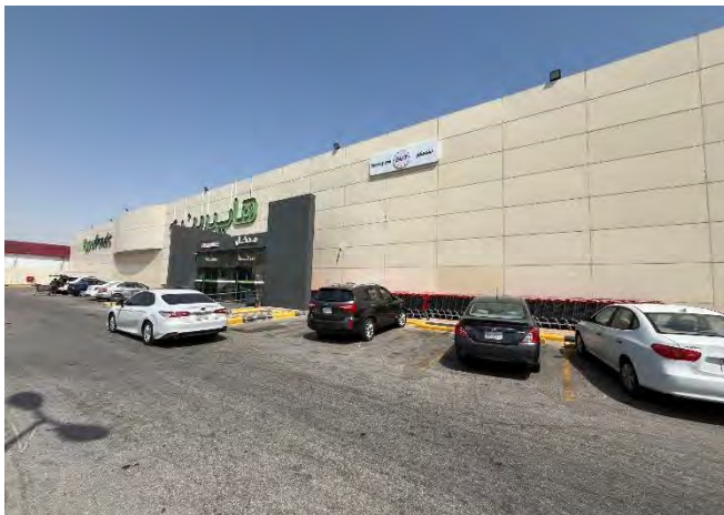
Source: JLL Inspection 2024
