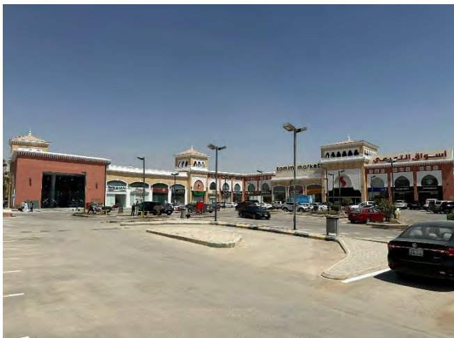
Source: JLL Inspection 2024
