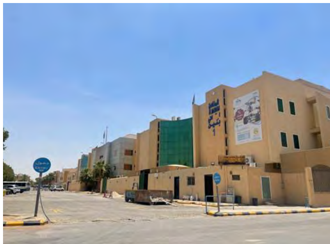
Source: JLL Inspection 2024
