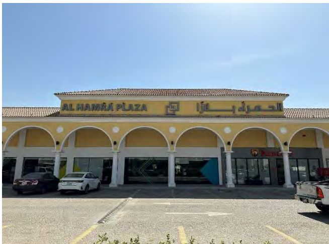
Source: JLL Inspection 2024
