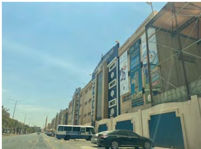
Source: JLL Inspection 2024
