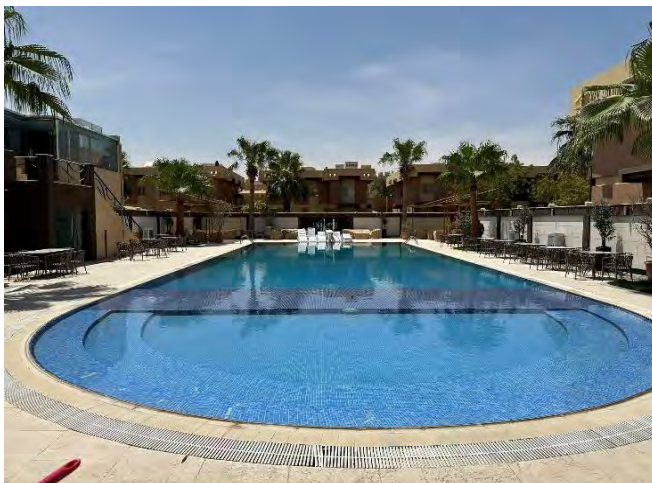
Source: JLL Inspection 2024
