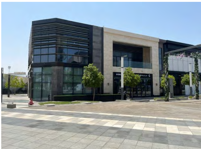
Source: JLL Inspection 2024
