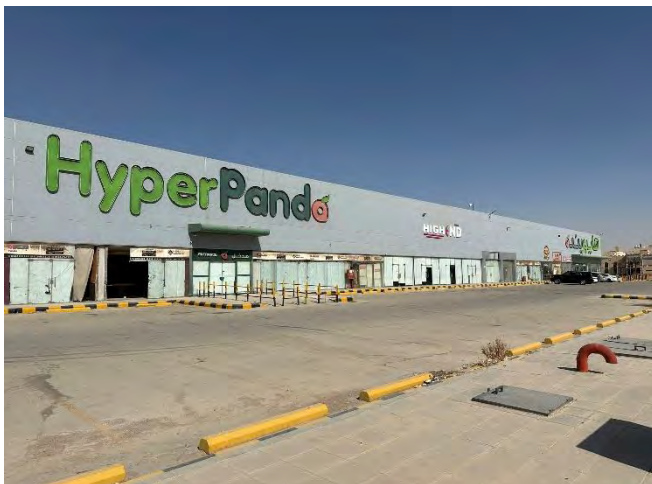
Source: JLL Inspection 2024
