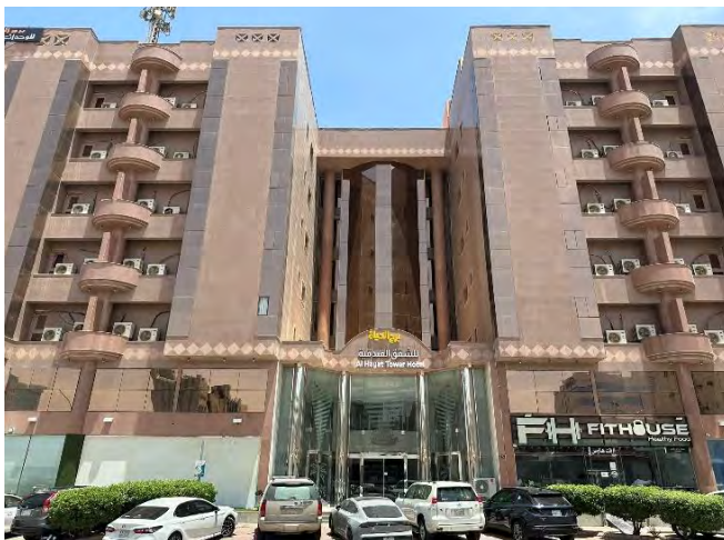
Source: JLL Inspection 2024
