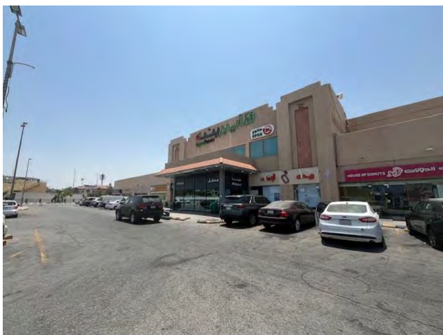
Source: JLL Inspection 2024
