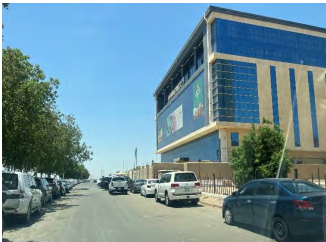
Source: JLL Inspection 2024
