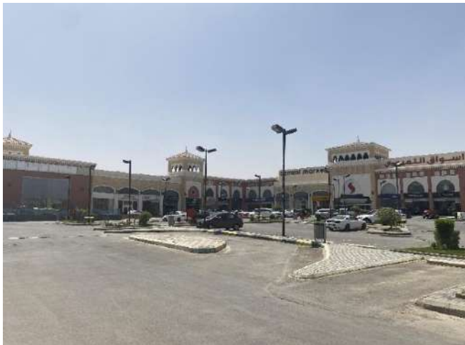
Source: JLL Inspection 2023
