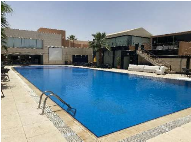
Source: JLL Inspection 2023
