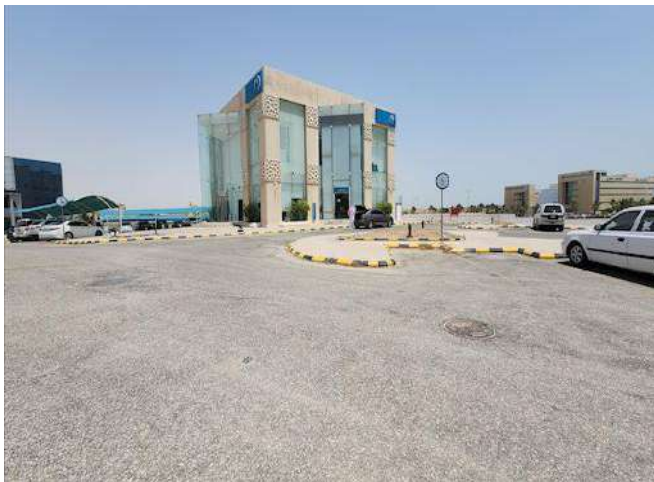
Source: JLL Inspection 2023
