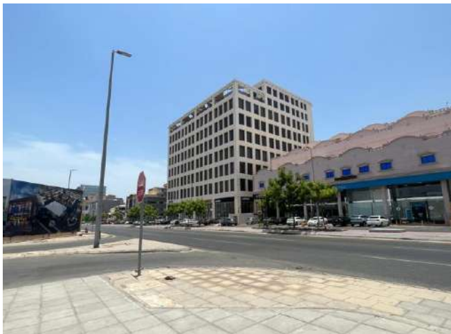
Source: JLL Inspection 2023
