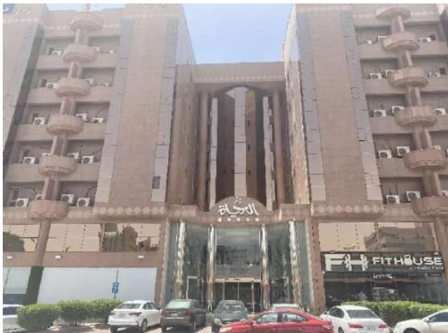
Source: JLL Inspection 2023
